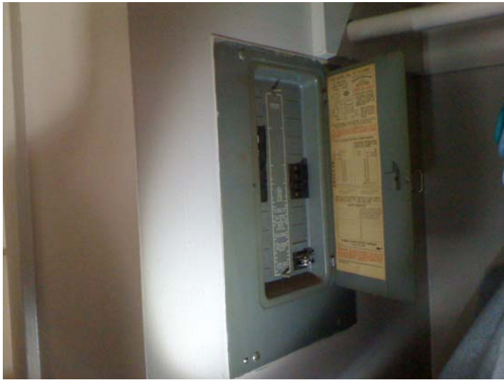
This is one of the FPE Stab-Lok circuit breaker panels, found in each apartment.
