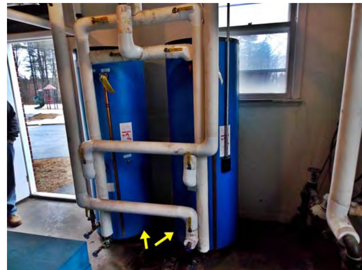
Each boiler room has a pair of insulated DHW storage tanks.
