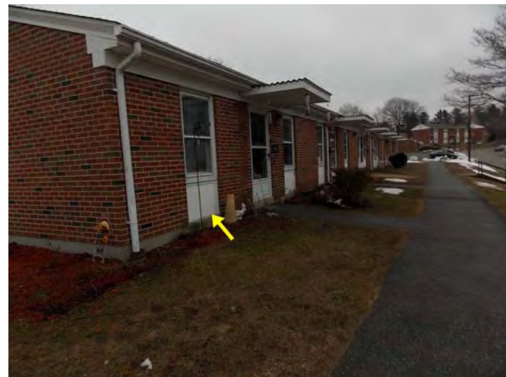
Buildings have brick exterior walls with vinyl window panels (arrow).
