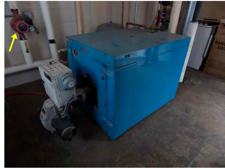
One of the oil-fired boilers used to produce hydronic heat and DHW. To the left (arrow) is one of the circulating pumps.
