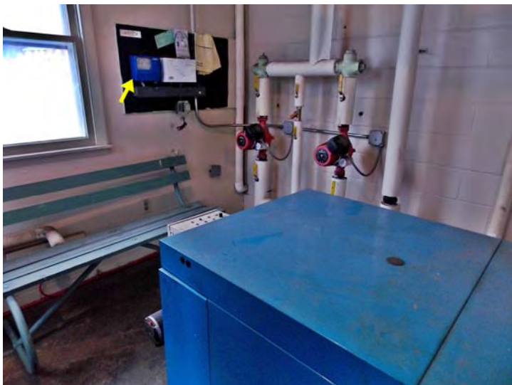
A view of the Tekmar controller (arrow).
